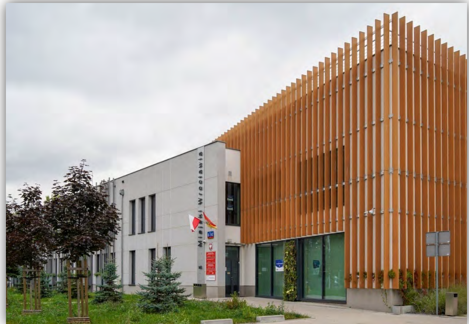
Environment and Agriculture Division building at Hubska str.
