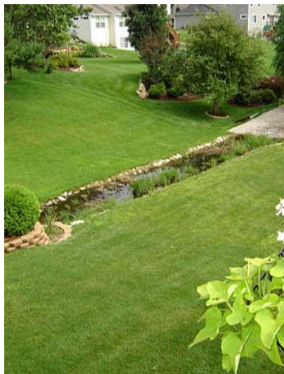
Reinforced Turf will Transport Significant Water Flows while Protecting against Erosion
